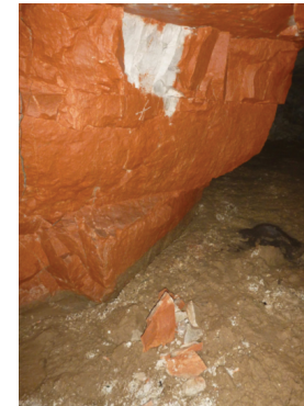
Surveillance visuelle © Cerema
